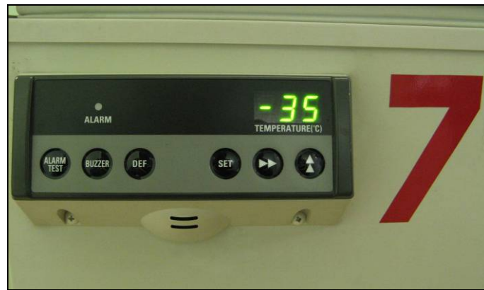
Fig 18.16-2. Control panel of the freezer showing it achieving -35C.
